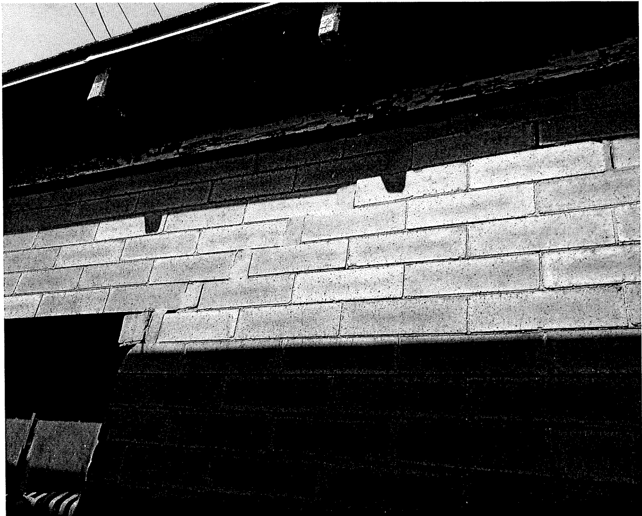
EAST WALL - NE PORTION UPPER VIEW
