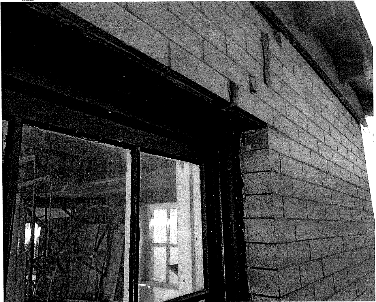
SOUTH WALL SE CORNER
