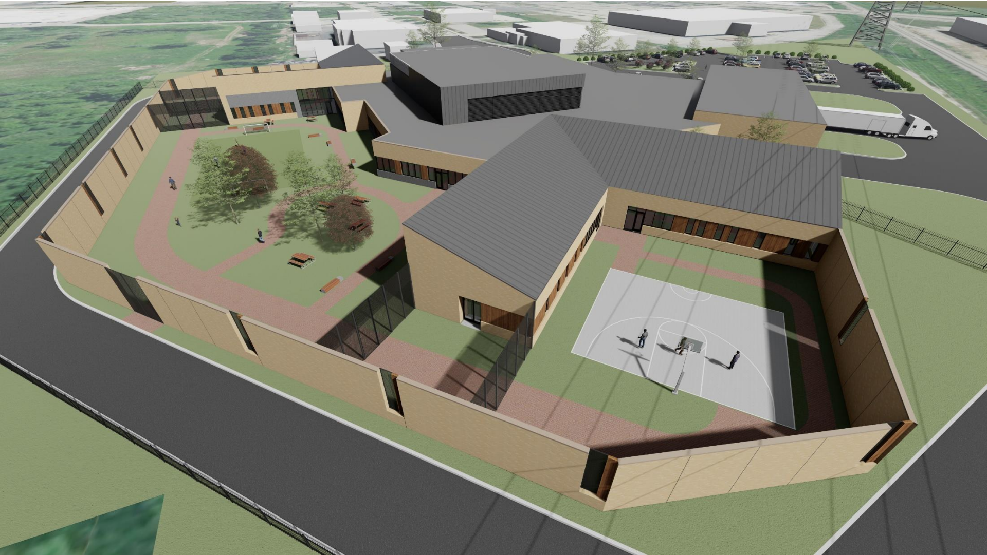
AERIAL VIEW FROM NORTHWEST
