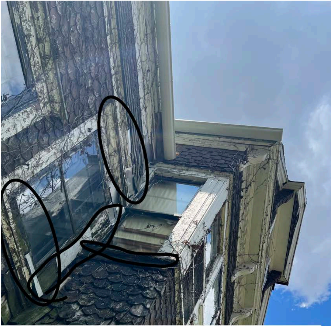
Replace window sills using cedar. Rebuild moldings to match using cedar.
