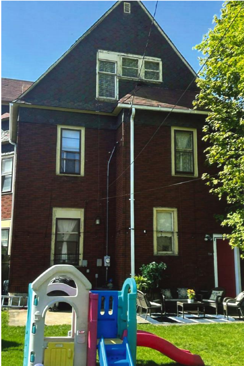
Northern (rear) façade to be restored
