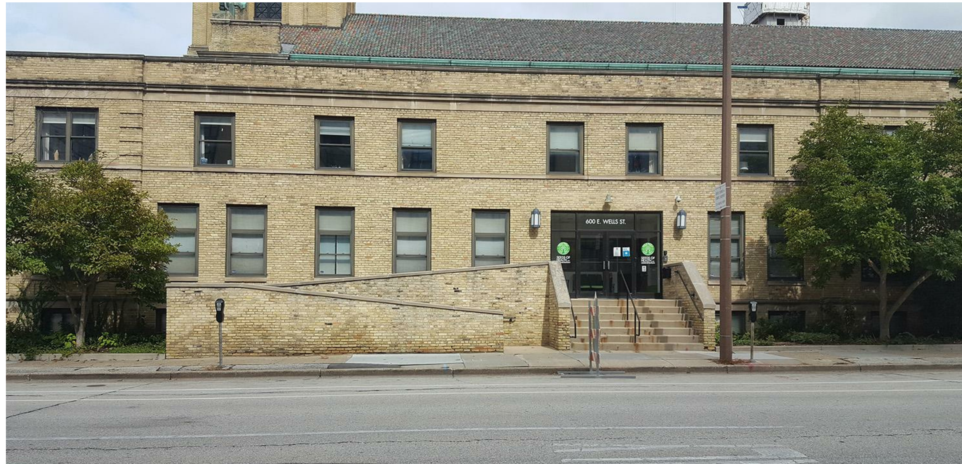
EXISTING PHOTO OF EAST ELEVATION.
