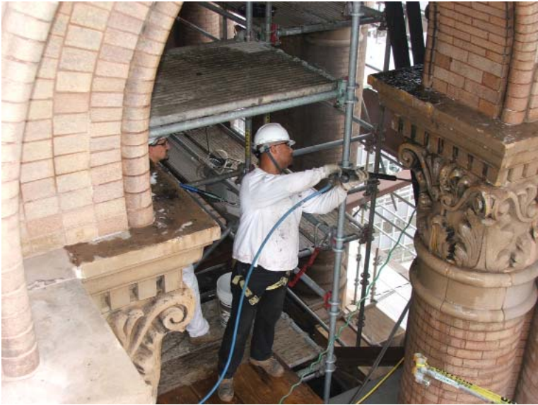
Image 3: Worker cleaning exterior brick. Image courtesy of UWM School of Architecture/ Historic Preservation Department
