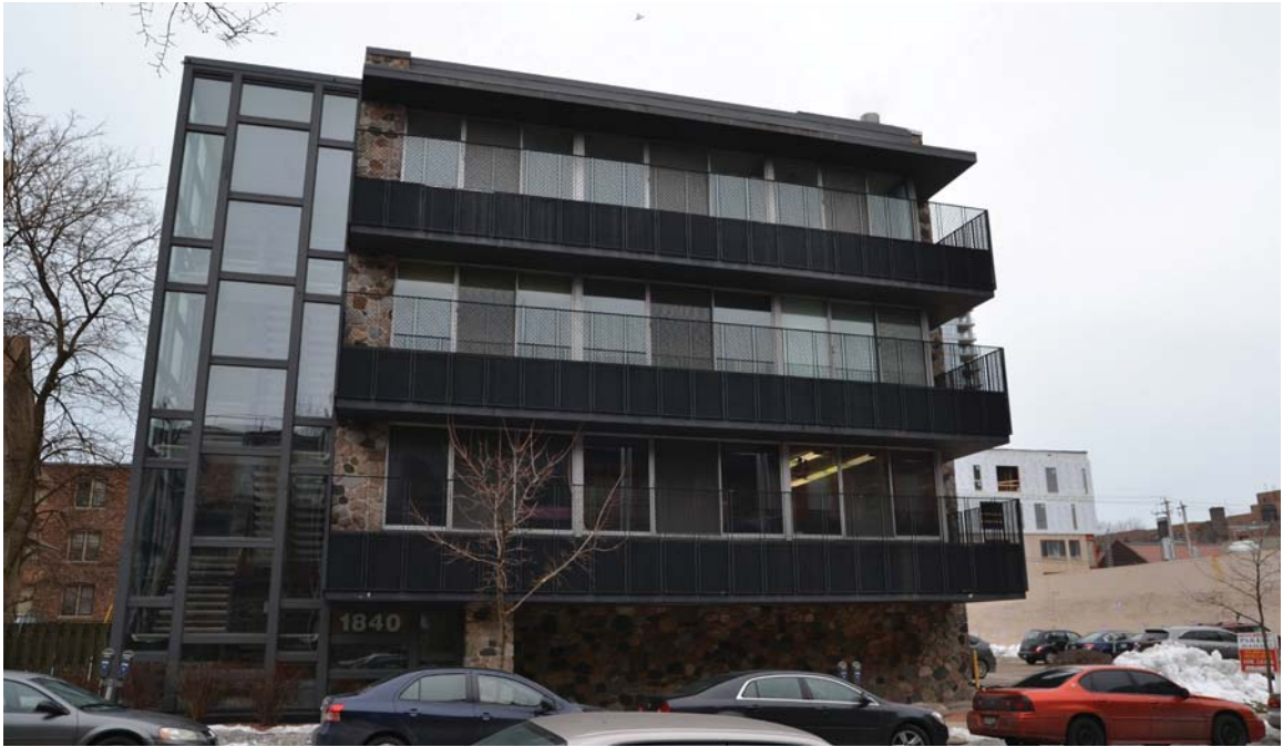
13. EXISTING BUILDING AT 1840 N FARWELL AVE
