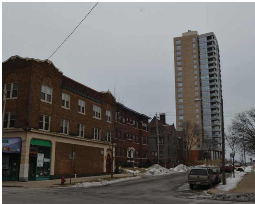
23. VIEW EAST ON FARWELL
