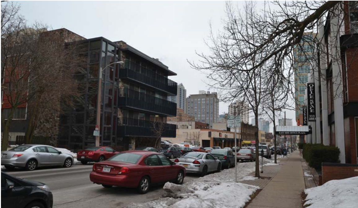
11. VIEW SOUTH ON FARWELL
