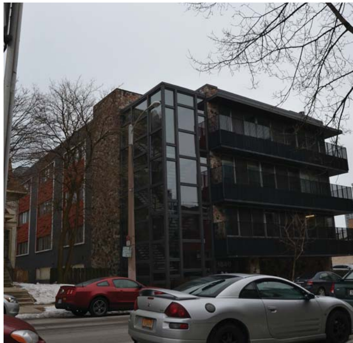
12. EXISTING BUILDING AT 1840 N FARWELL AVE
