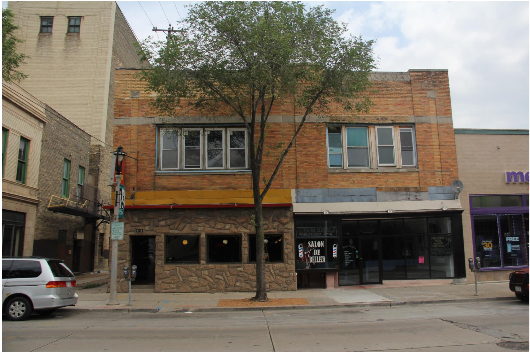
Current condition of façade 2016.
