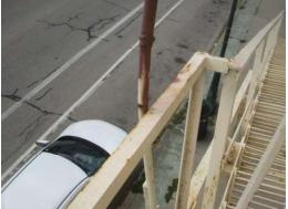
The counterweight system worked properly, except for the interference of the bent rod (see above). The stairs lowered at an appropriate pace and raised back up with minimal assistance once weight was removed.
