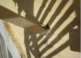
The staircase to the second-floor landing also shows some deterioration and rusting due to exposure to the elements. Some of the hardware attaching the treads to the rest of the structure are also rusted.
