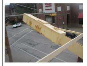
There is observed deterioration and rusting on the final flight of stairs as well. The hardware also shows deterioration.
