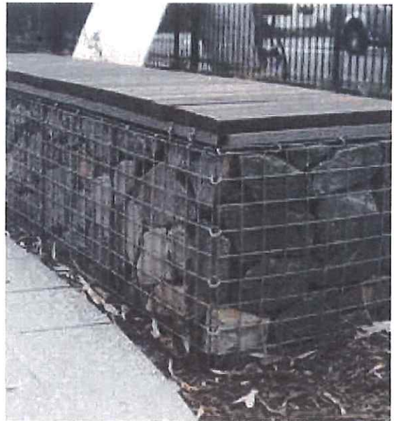
Gabion benches with Ipe wood tops (wax cut edges, unstained). Typical dimensions (18" H x 18" W x 6' L). WWM with max 4" openings. Typical limestone or fieldstone fill with max 6" dimension. Provide samples of all materials prior to construction.
