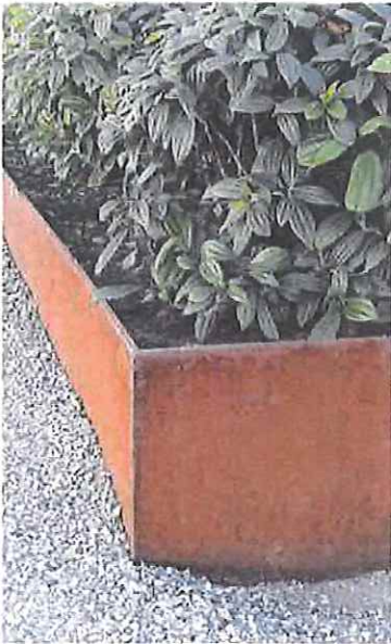
CorTen steel edging around all perennial beds. Minimum 14 Gauge thickness. 8" above finished grade errand perennials. 3" above grade between lawns and compacted limestone areas. Provide samples of all materials prior to construction.
