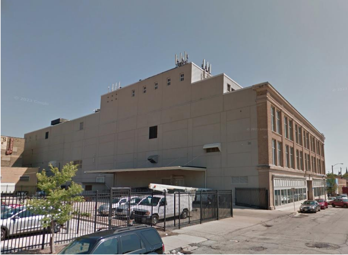
North façade, facing southeast
