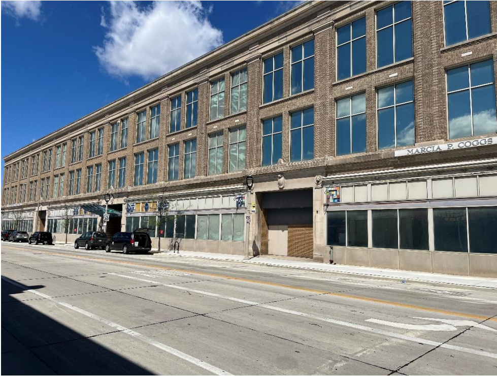
View looking west from W. Vliet Street.
