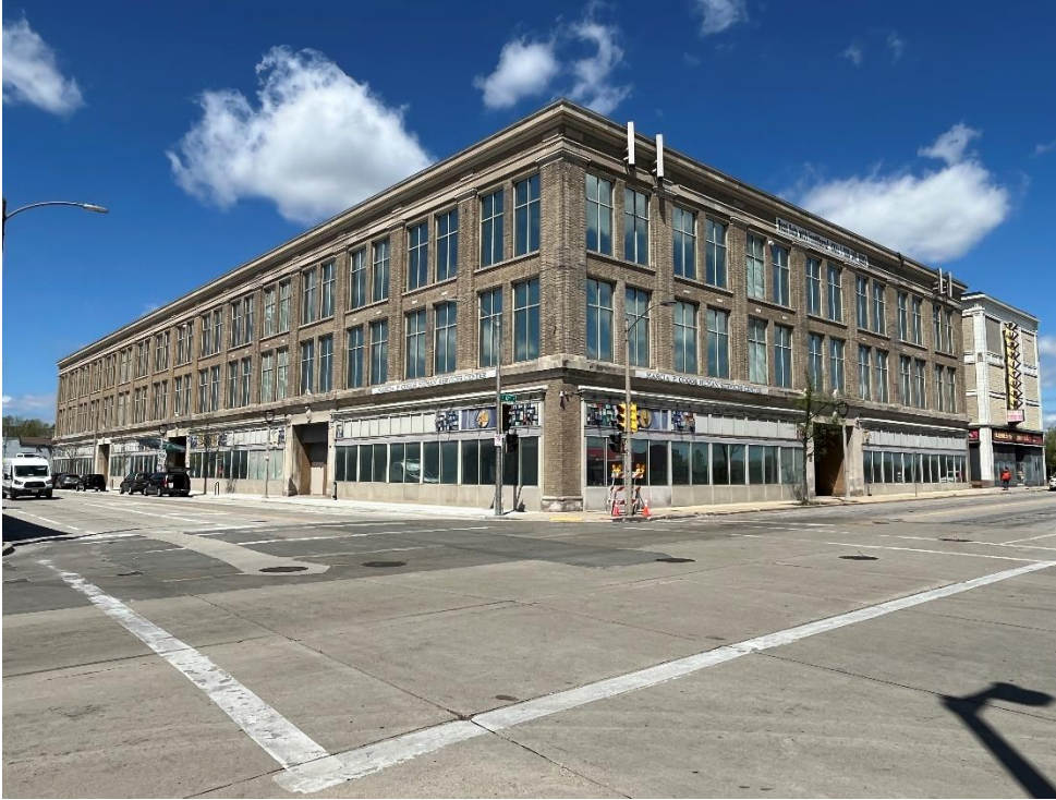
View looking northwest from W. Vliet Street.
