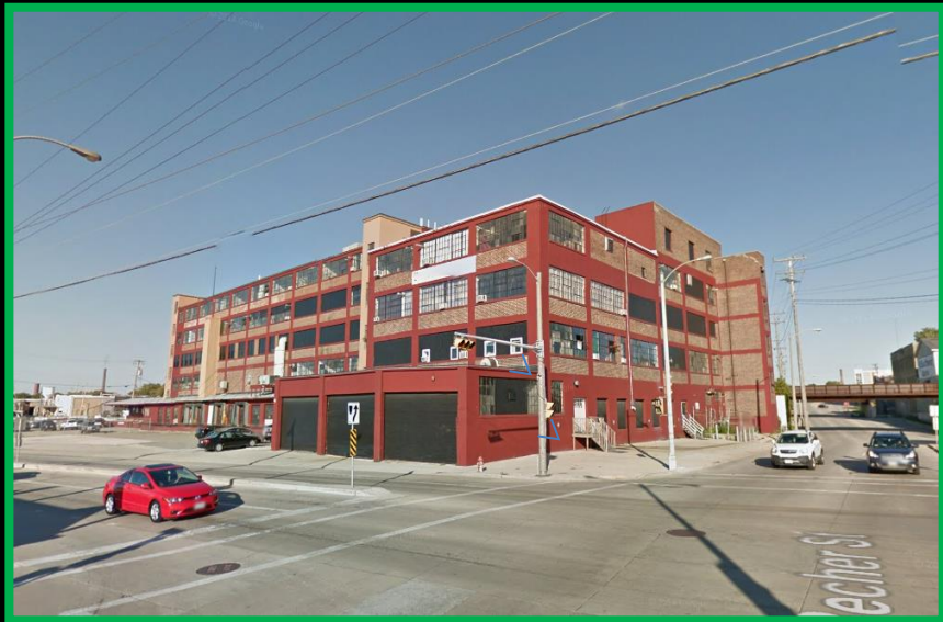
View from South 1st Street and West Becher Street
