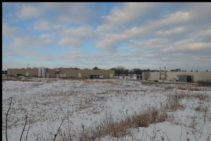
Looking north from the southern edge of property, toward location of building expansion.
