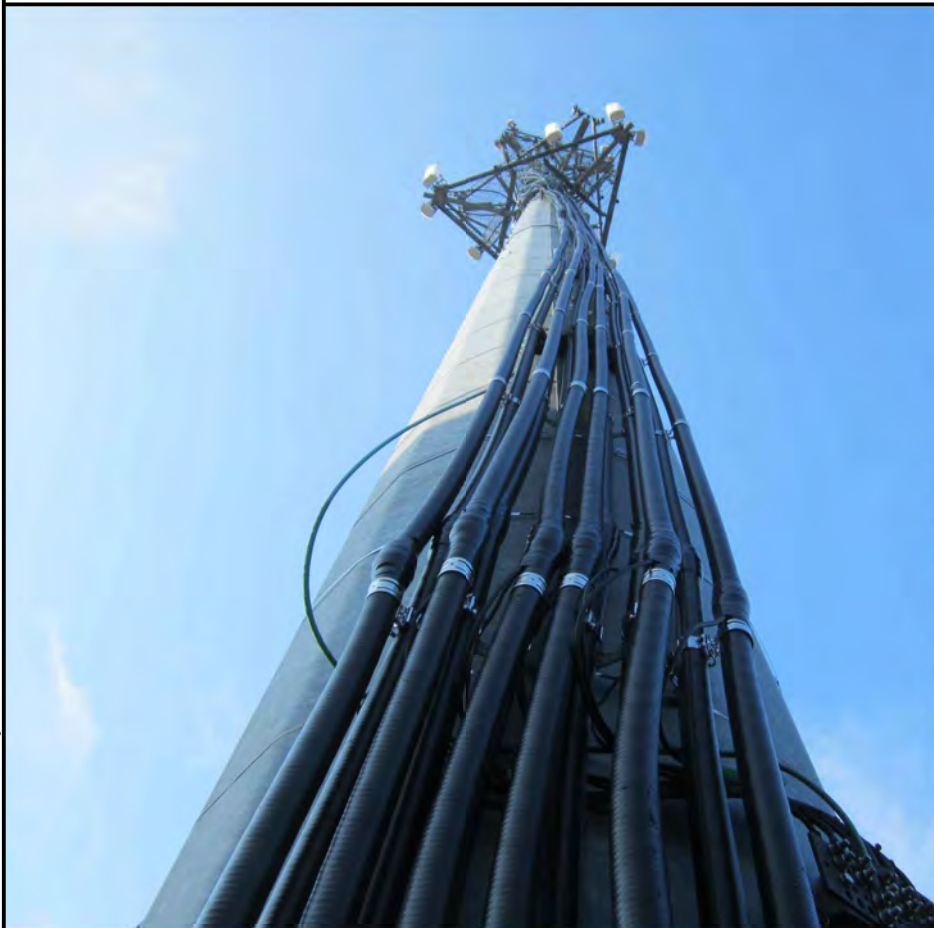
EXISTING TOWER SOUTHEAST FACE
