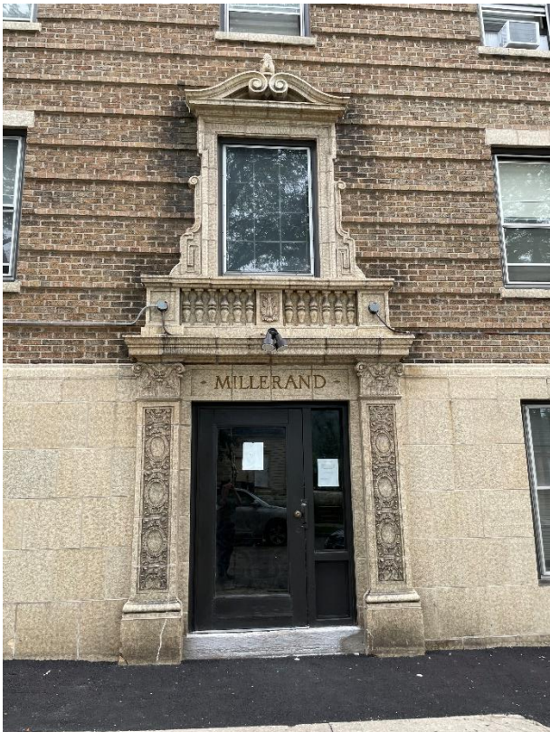
Details of secondary entrance on N. 31 st St.
