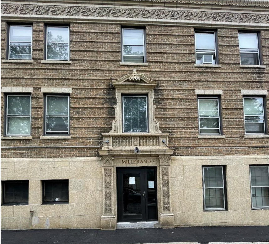
Details of west facade
