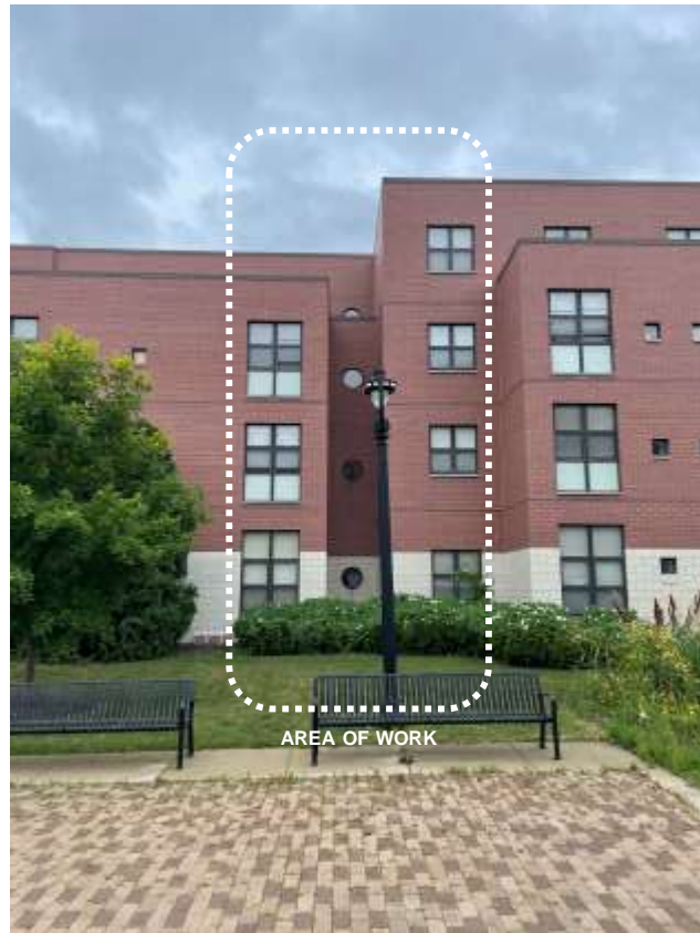
EXISTING WEST WING
