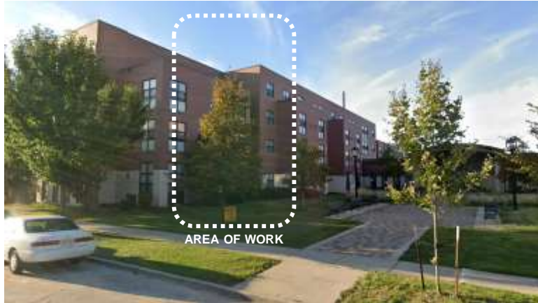
EXISTING WEST WING
