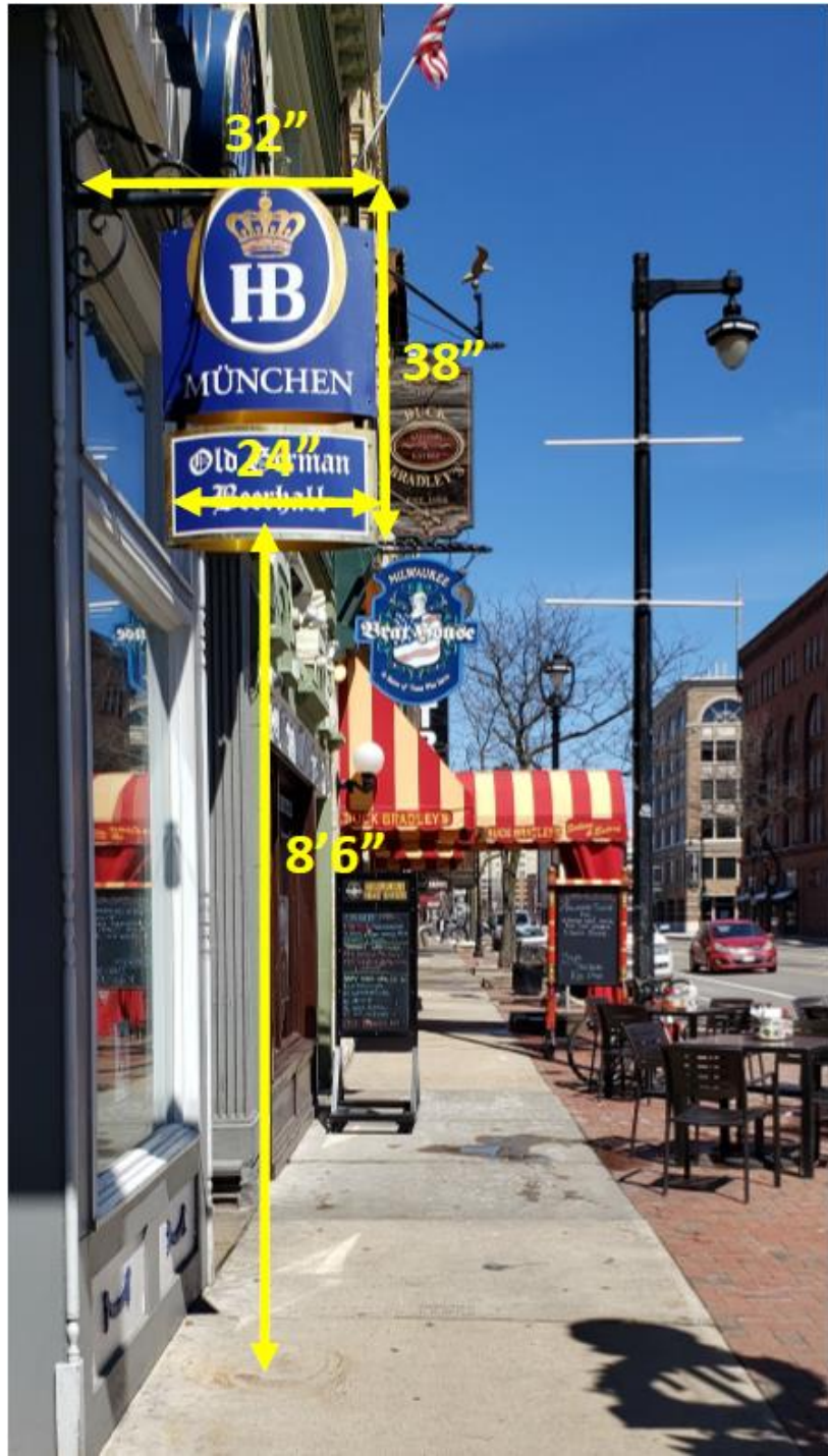
Annotated photo detailing the projection distance and height of the existing blade sign.
