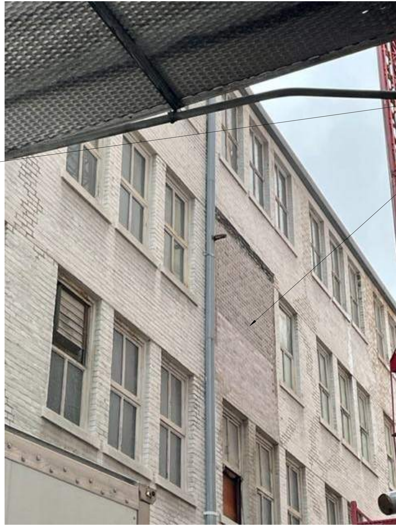
NORTH-EAST SKYBRIDGE INFILL
