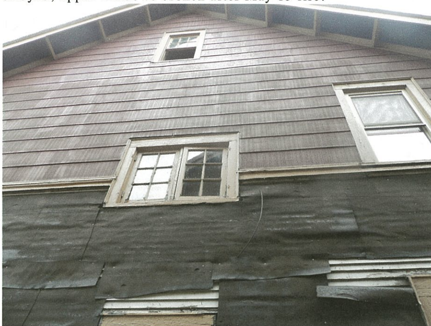
Figure 9: Casement, original double hung, and vinyl replacement windows (north elevation).
