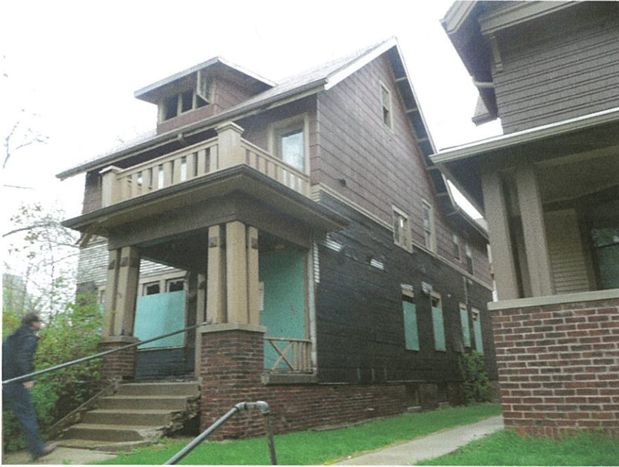
Figure 2: Front porches and north elevation.
