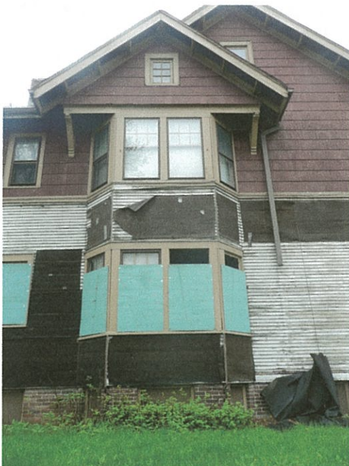
Figure 6: South elevation bay with integrated end-gable and roof supports.
