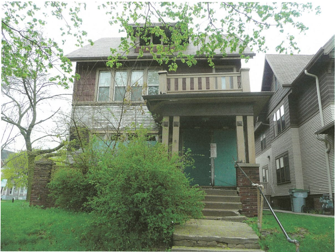
Figure 1: East elevation and front porches from 33rd Street.
