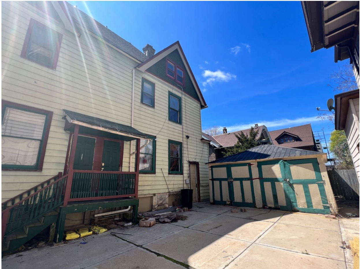
E7 - North Elevation of 2902-04 W State St, facing southwest
