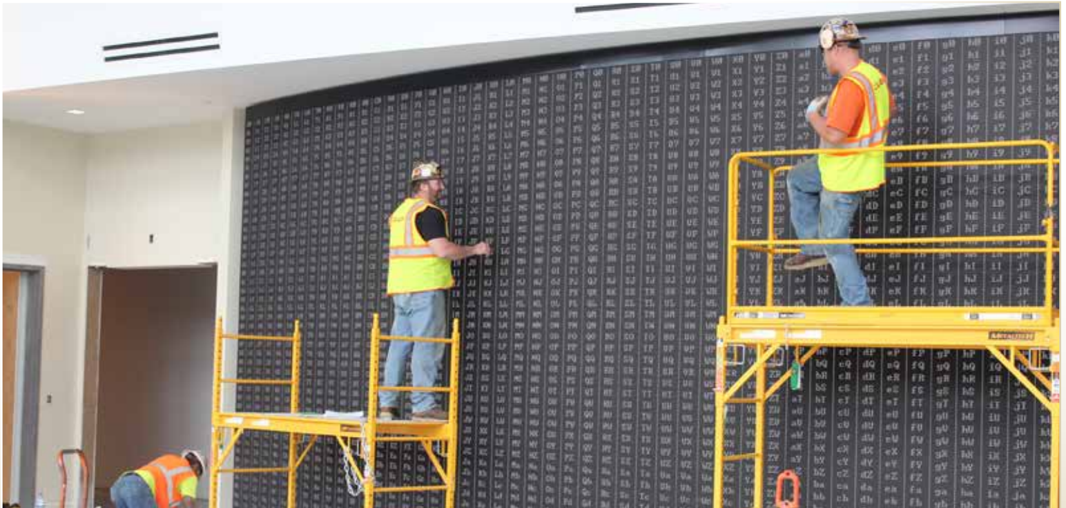
Worker installing display panels at the entrance lobby of the arena.
