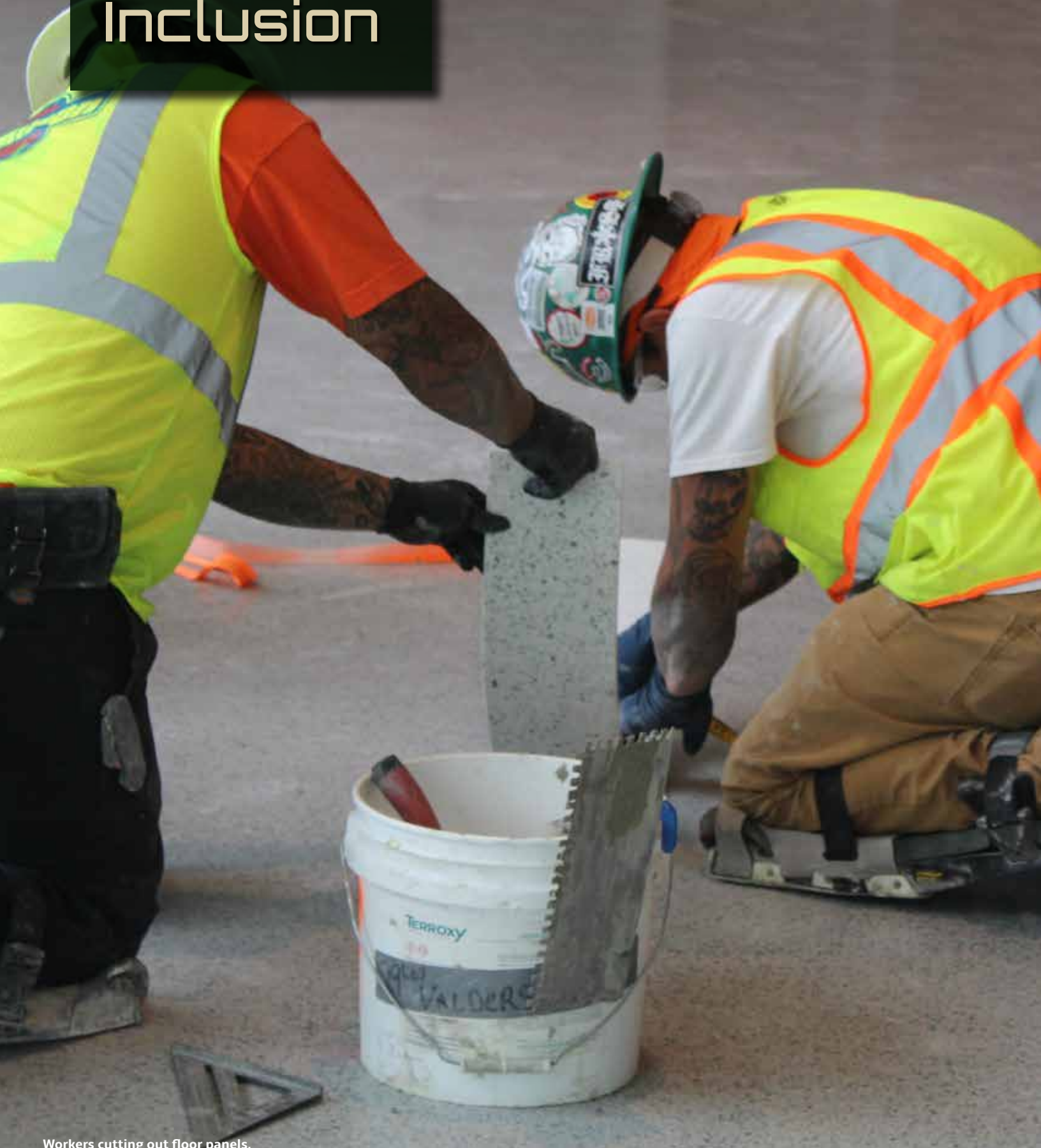
Workers cutting out floor panels.
