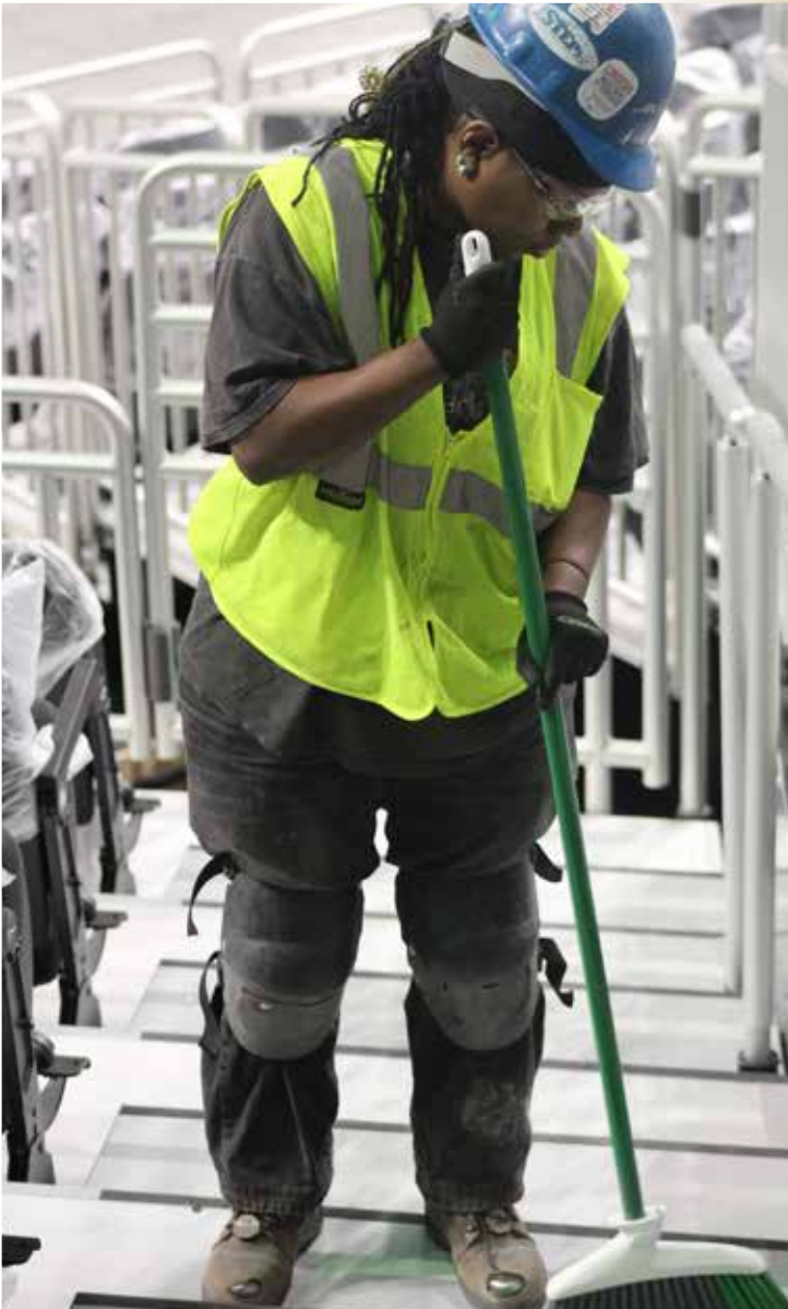
Worker sweeping after seats installation.
