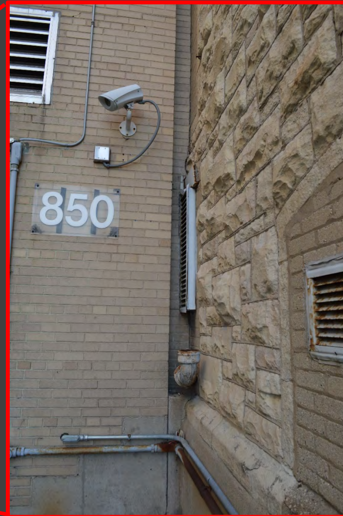
PARISH HOUSE ADJACENT TO ANOTHER BUILDING
