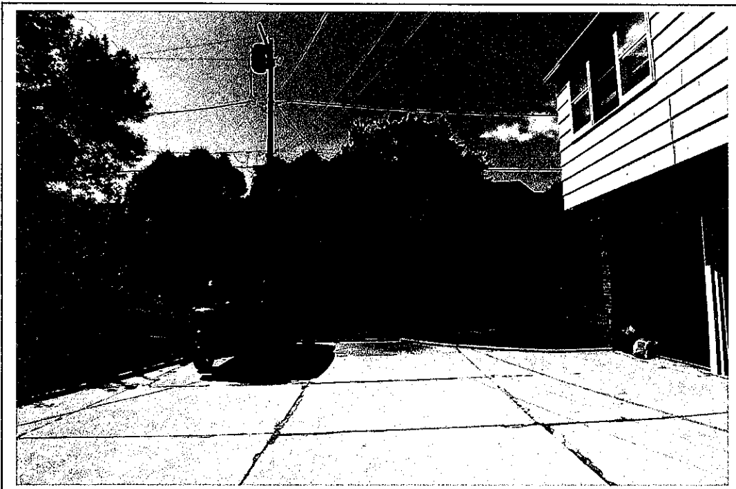
Driveway to be replaced with new concrete, brick border and curb, and brick inlay pattern.
