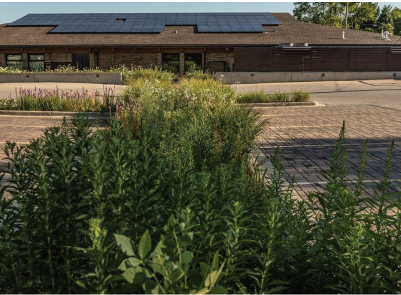
▲ Example of bioswales and permeable paving at Tippecanoe Library. Source: Urban Milwaukee
