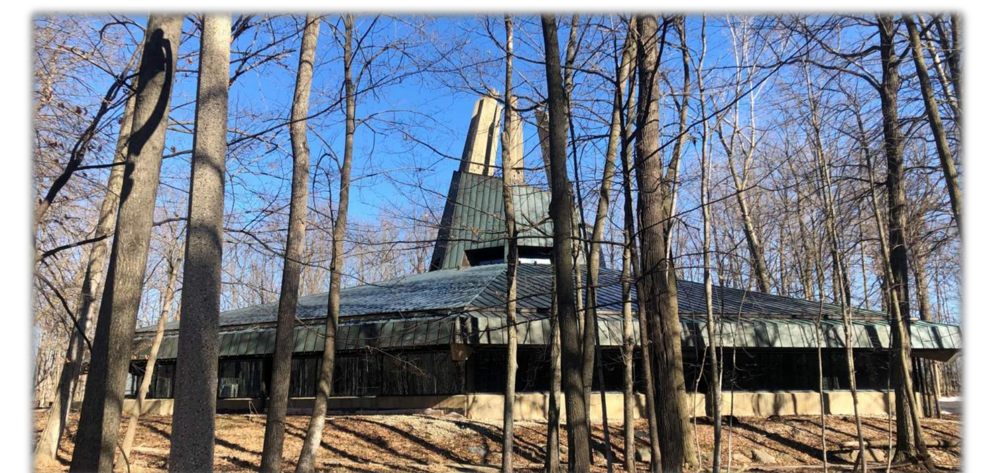
Vacant Existing Building along Northeast Portion of the Site
