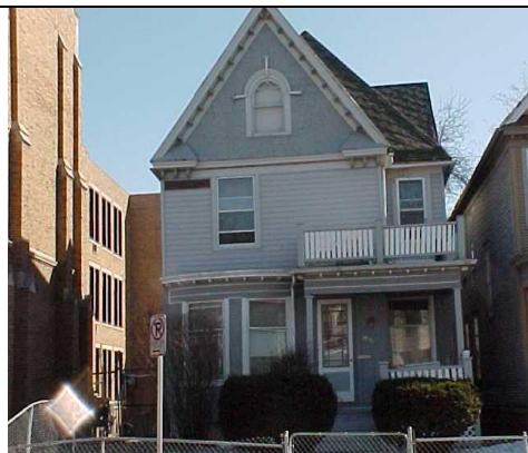
Parcel #7 1930 North 36 th Street
