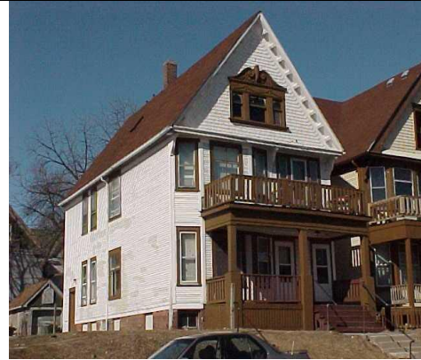
Parcel #2 1909-11 North 35 th Street
