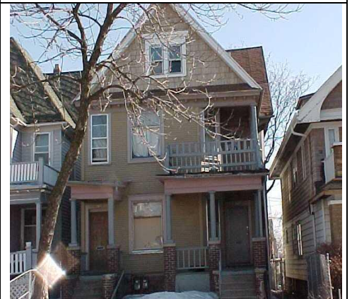
Parcel #6 1924-26 North 36 th Street
