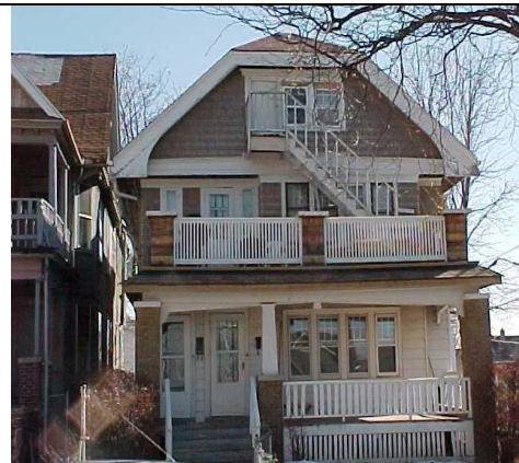
Parcel #5 1920-22 North 36 th Street
