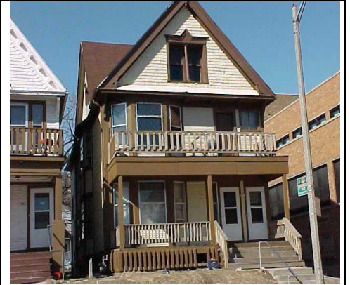
Parcel #3 1913-15 North 35 th Street
