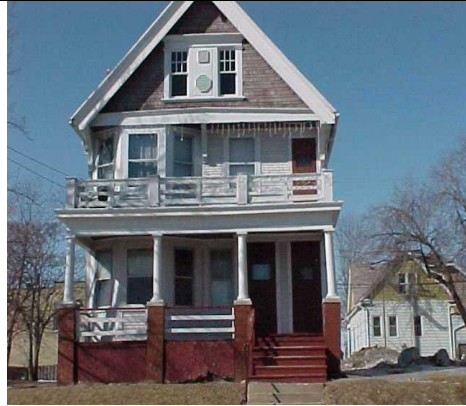
Parcel #1 1849-51 North 35 th Street
