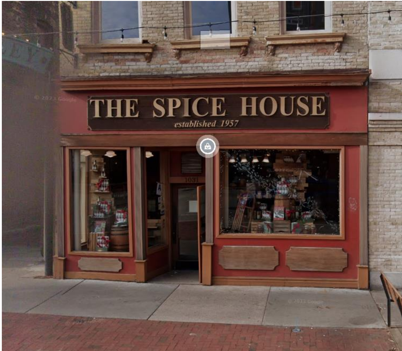
Storefront to be painted black with tan trim, plaques to be painted white with tan trim
