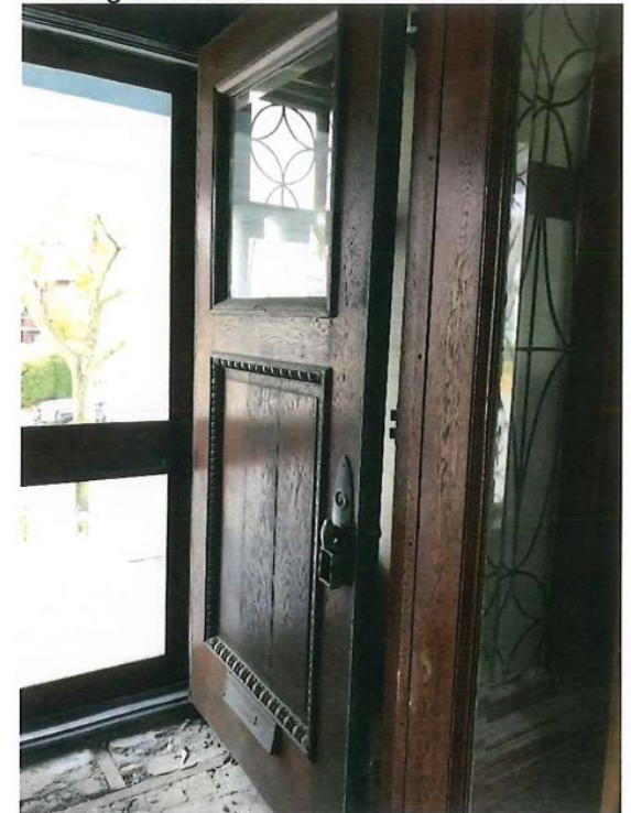
Existing Front Door
