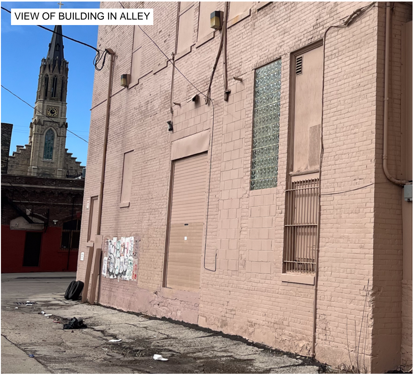
HIGHLIGHTED AREA IS COILING OVERHEAD DOOR TO BE REMOVED AND INFILLED.
