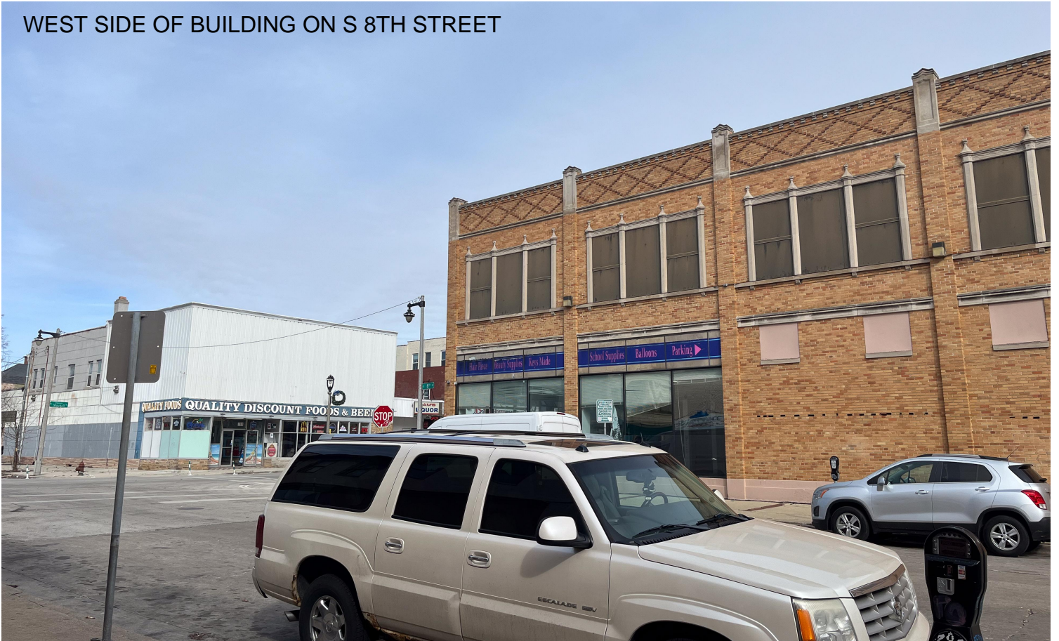
WEST SIDE OF BUILDING ON S 8TH STREET
