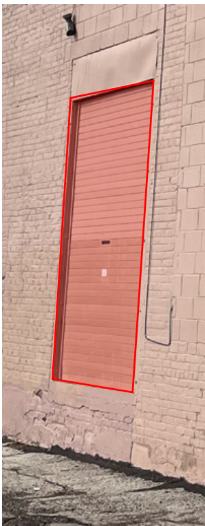
HIGHLIGHTED AREA IS COILING OVERHEAD DOOR TO BE REMOVED AND INFILLED.
