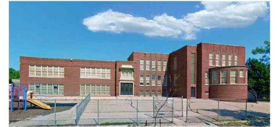
EXISTING WEST FACADE AND SMALL PLAYGROUND
