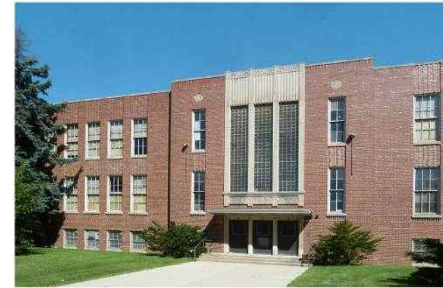
EXISTING FRONT ENTRY OF SCHOOL (SOUTH)
