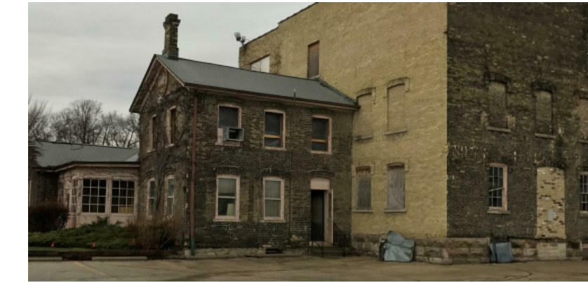
6 CURRENT CONDITIONS (PHOTO FROM THE REVISED HISTORIC DESIGNATION STUDY REPORT) 1/12" = 1'-0"
