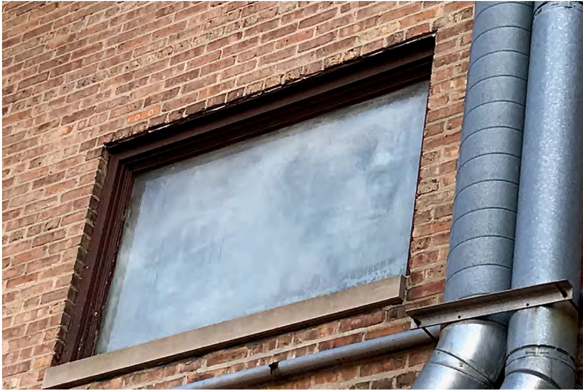
IMAGE 23: Closer view of typical window unit conditions. Preserve, LLC 2021.
