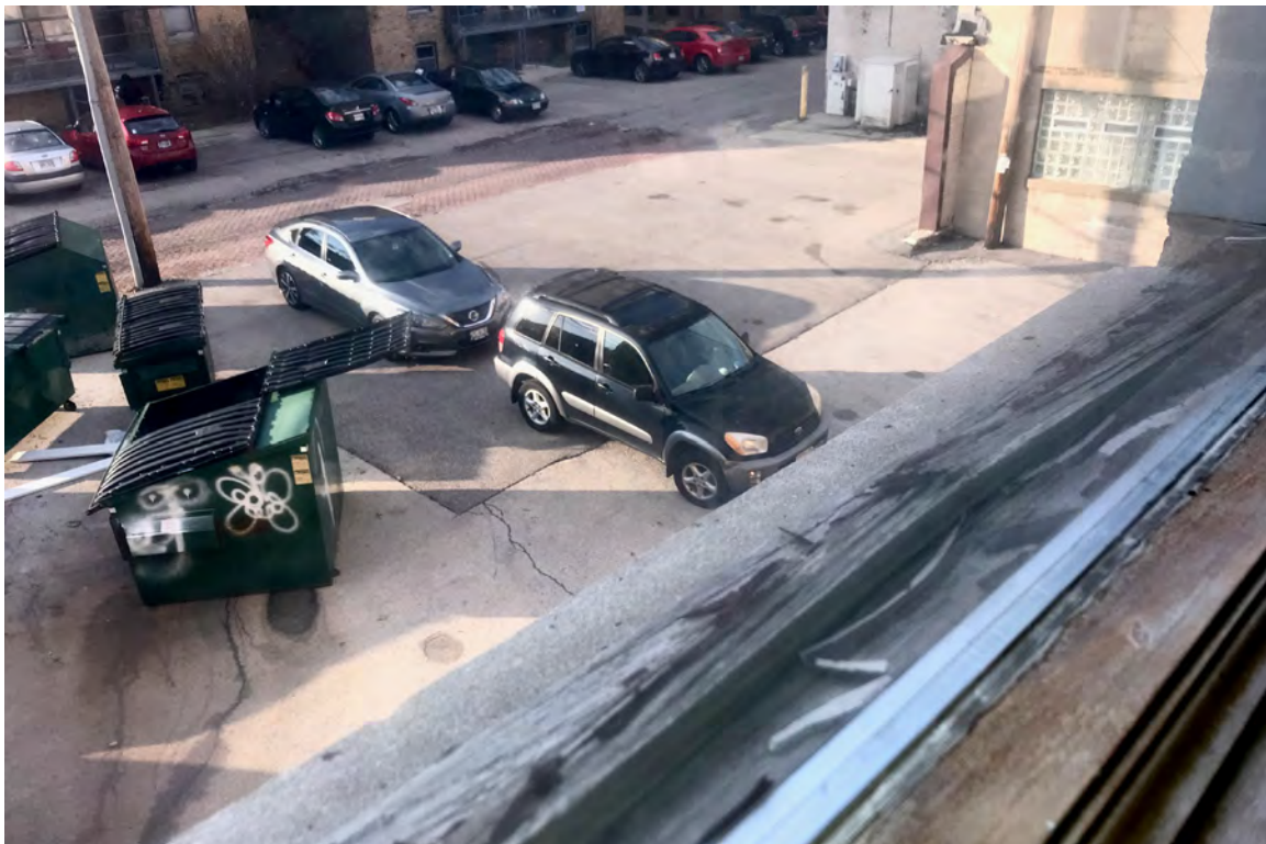
IMAGE 30: View of blown-out sill due to active moisture at window units on west elevation. Preserve, LLC 2021.
