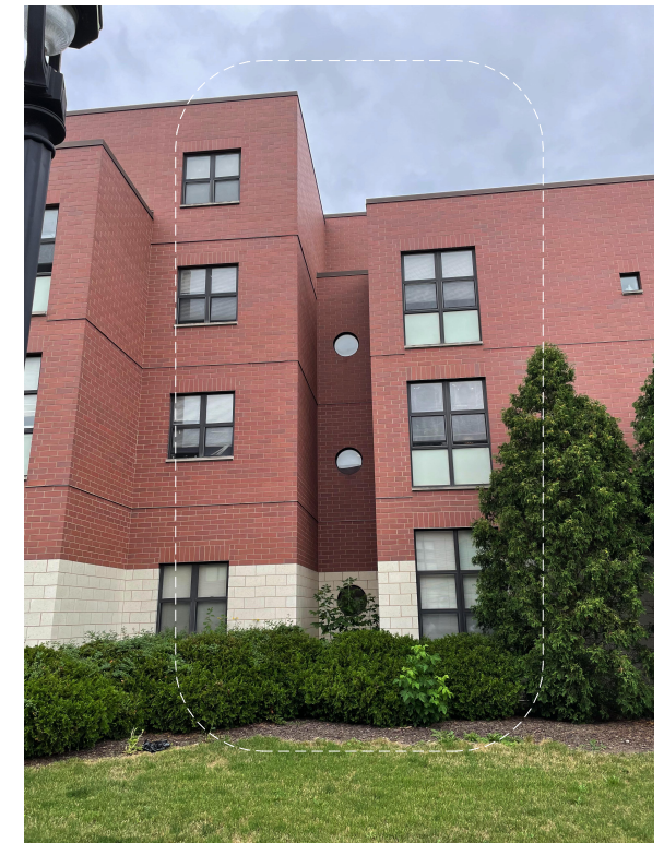
EAST WING - AREA OF WORK
