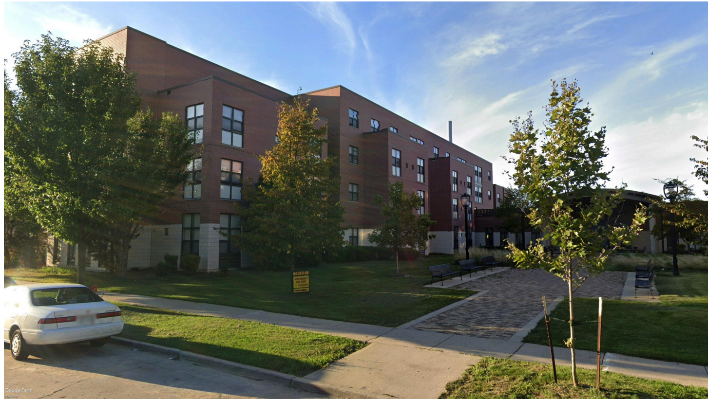
EXISTING WEST WING
