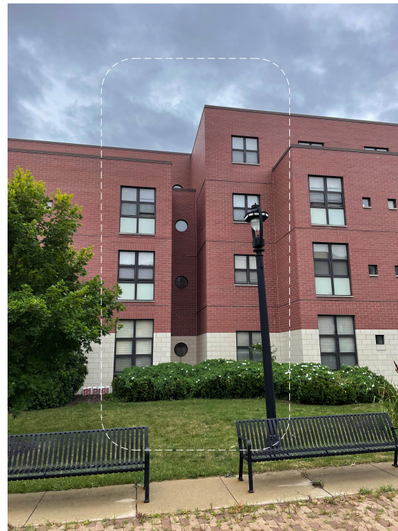
WEST WING - AREA OF WORK
