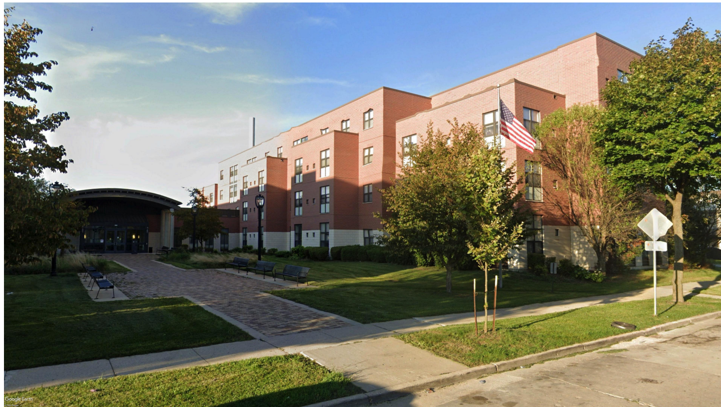
EXISTING EAST WING
