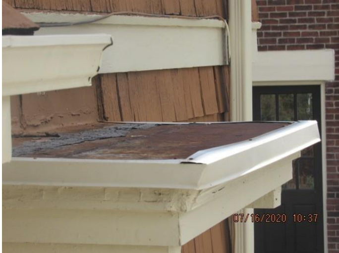
Typical built-in gutter and secondary roof conditions.
