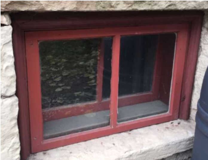
Example of existing 2-pane exterior storm windows on basement
