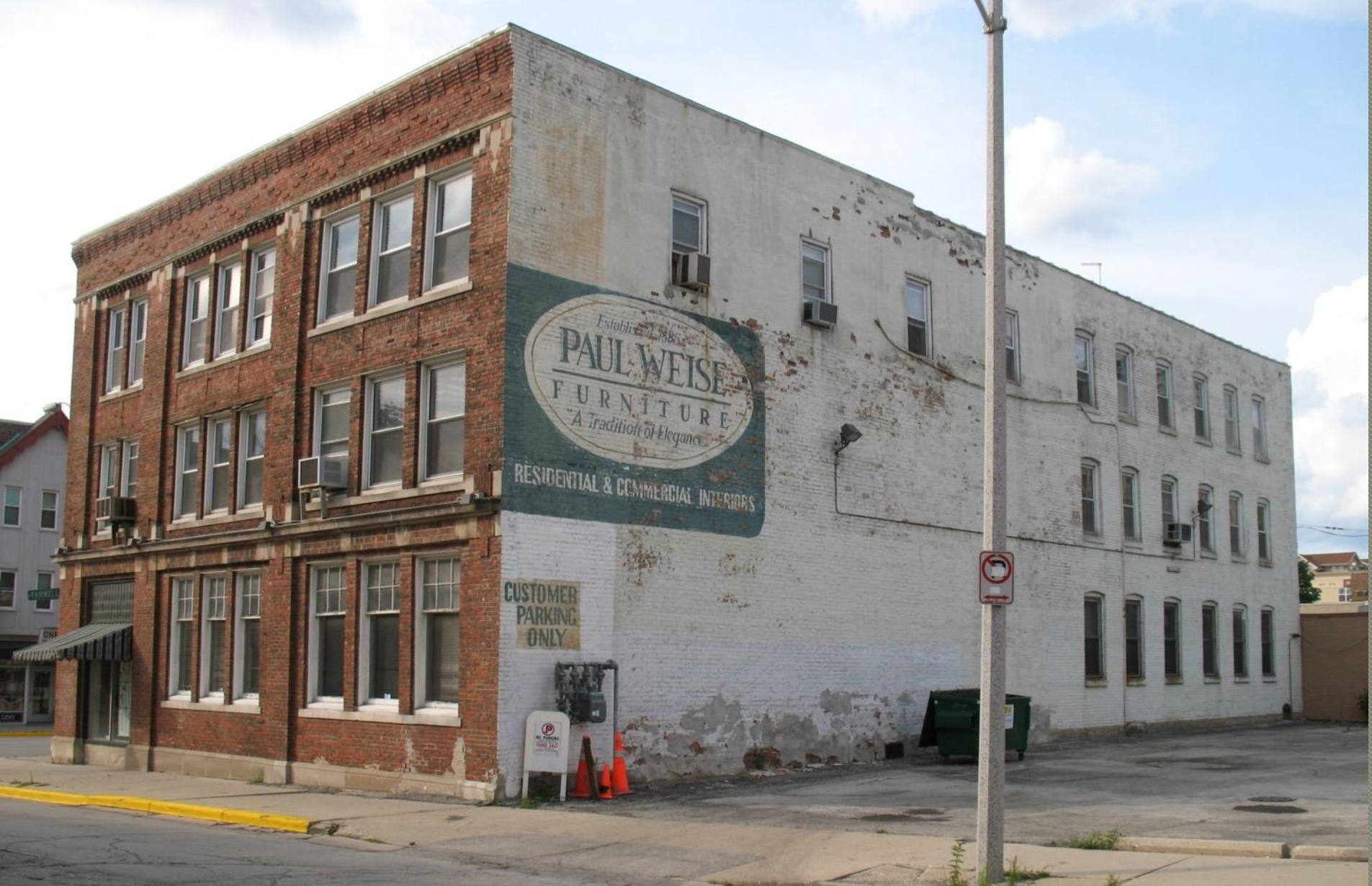
East Elevation showing painted and parged brick and ghost sign
