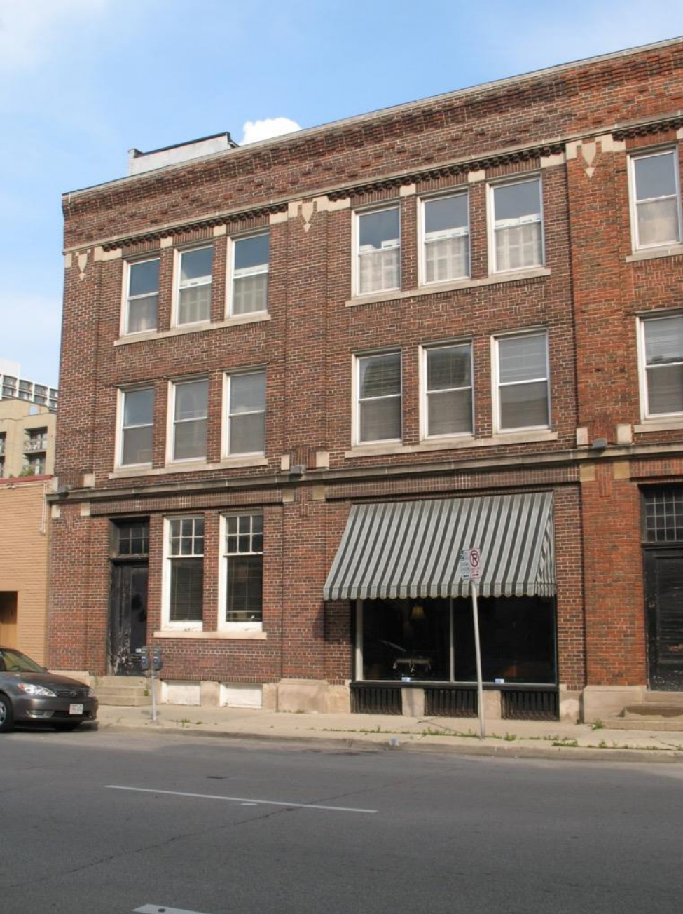
Note 1922 addition has slightly different color brick
