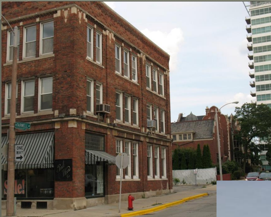
Elizabeth Black House on Prospect Avenue built in 1901 just east of the Eschweiler shop
