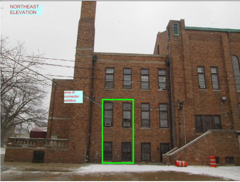
Point of connection. These 4 windows will be removed. Perspective view, looking south along Teutonia.
