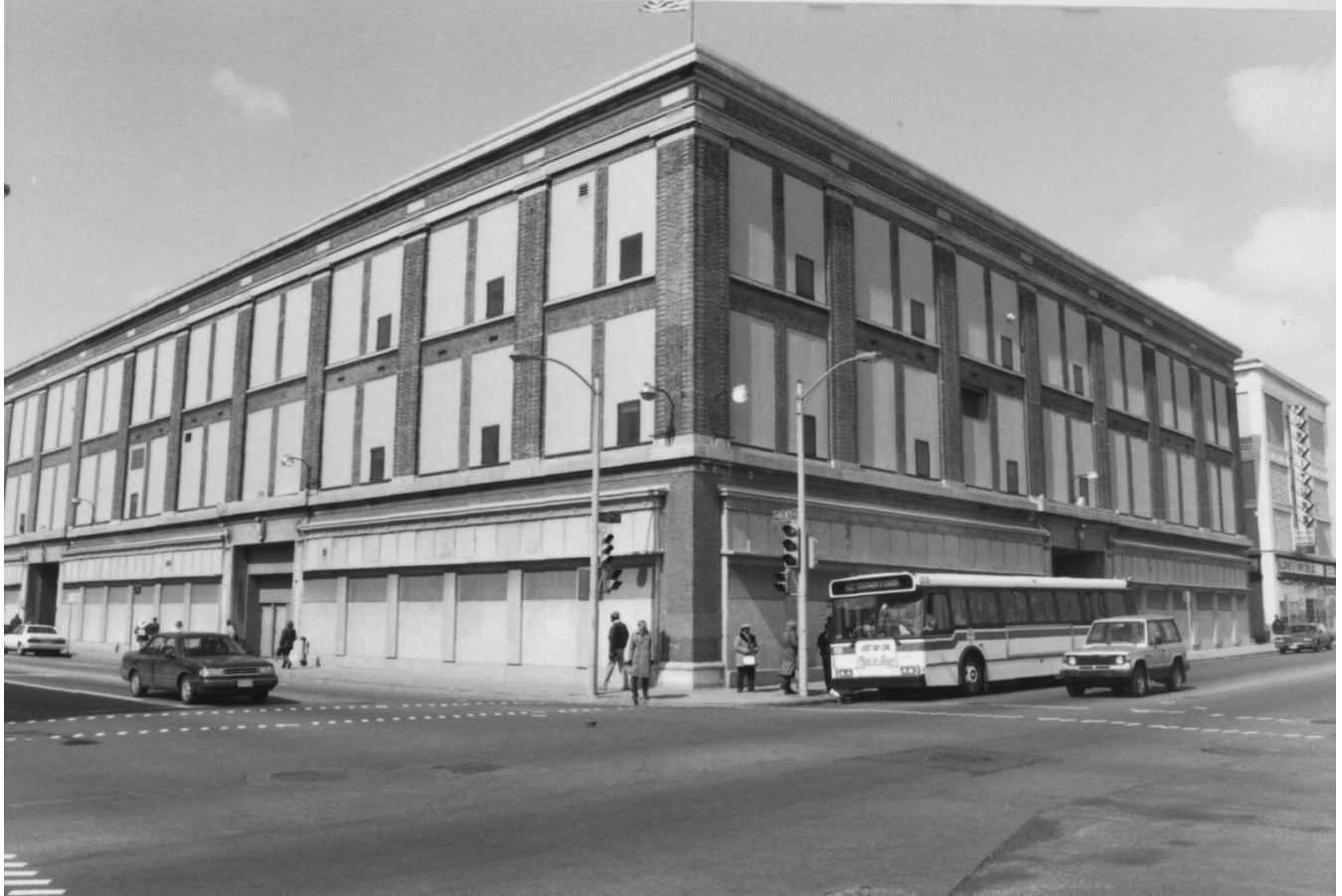
Figure 10. Wisconsin Architecture and History Inventory, Record #78966. Photo taken 1993. Storefront windows on first floor and windows on upper levels had been infilled. By 1993, decorative parapet had been removed.
