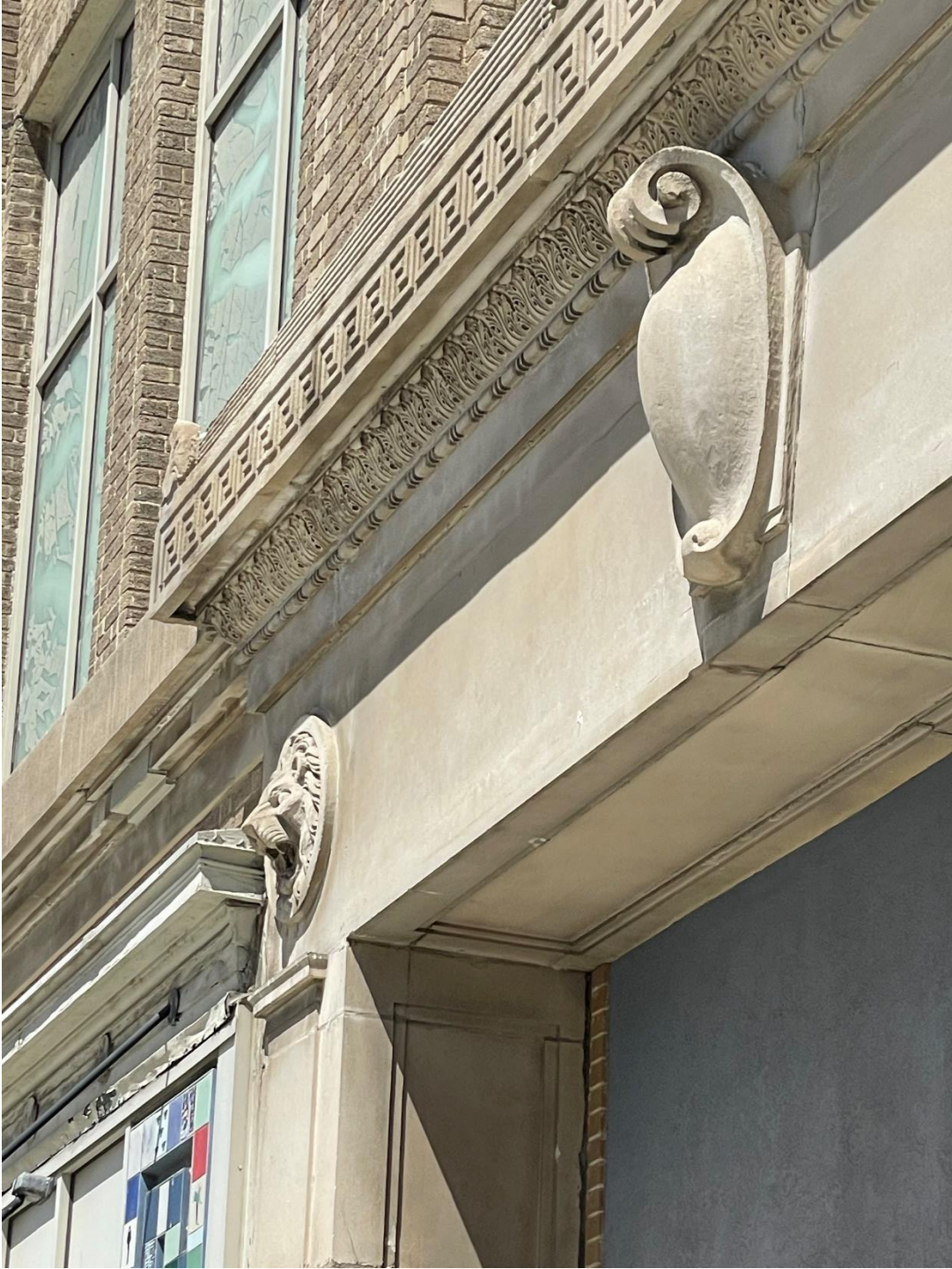
Close up of entrance detailing
