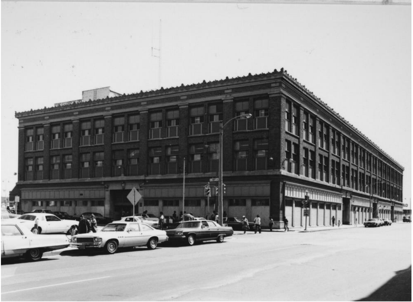
Figure 9. Wisconsin Architecture and History Inventory, Record #78966. Photo taken 1979. Looking northwest
