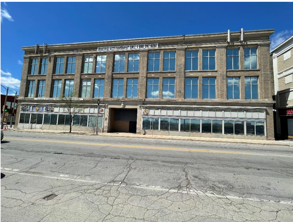
East façade, view looking west from N. 12 th Street.
