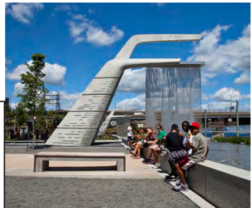
Artistic water fountain in Toronto, Canada that filters water and is part of a neighborhood-wide stormwater treatment facility.
