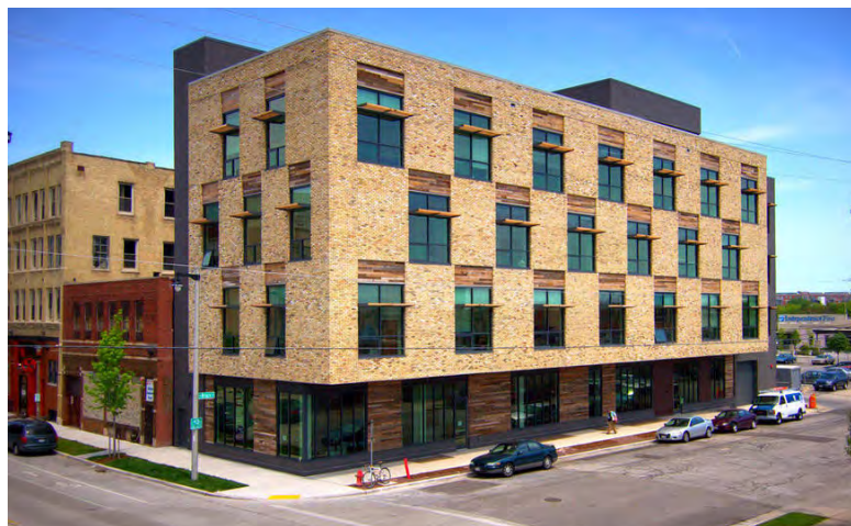
The Clock Shadow Building in Walker's Point demonstrates context sensitive development that contributes to a walkable environment.
