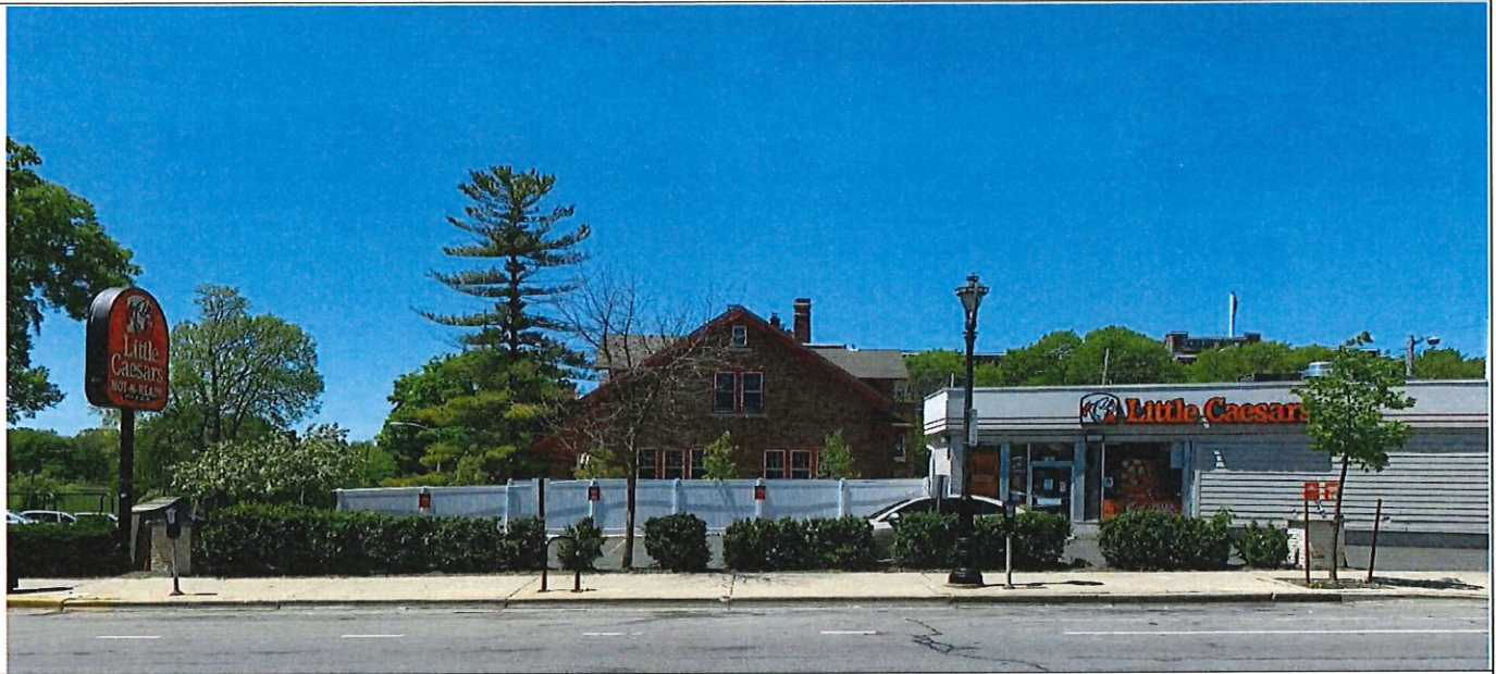
Facing West Across Oakland Avenue
