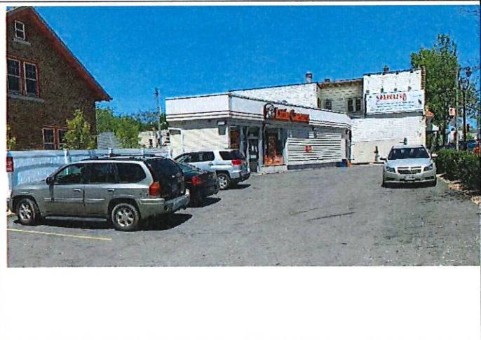
Across Parking Lot Facing North
