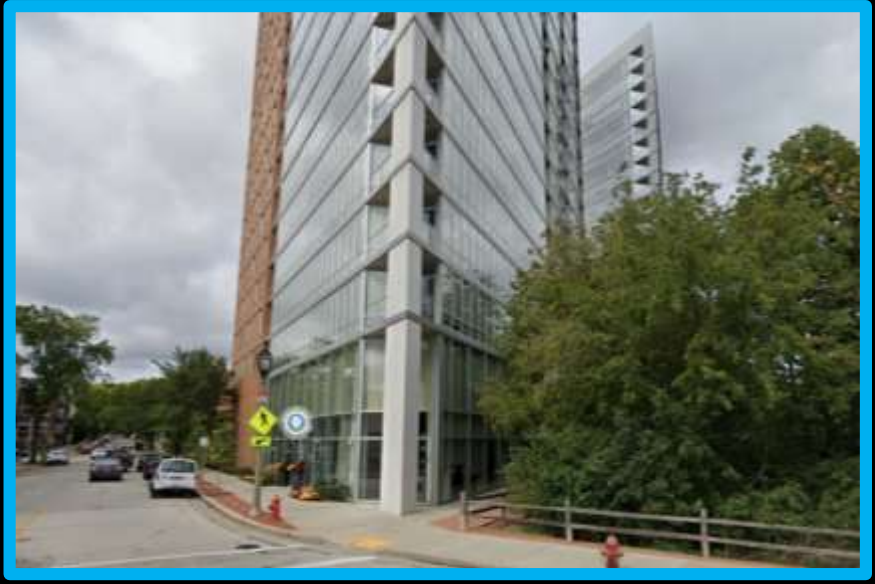
View from East Lafayette Place looking north
