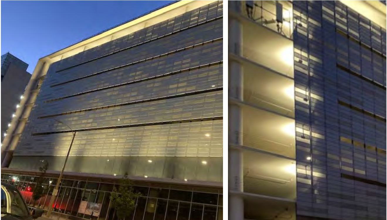
Lighting example for painted cast-in concrete (7SEVENTY 7 garage photos)
