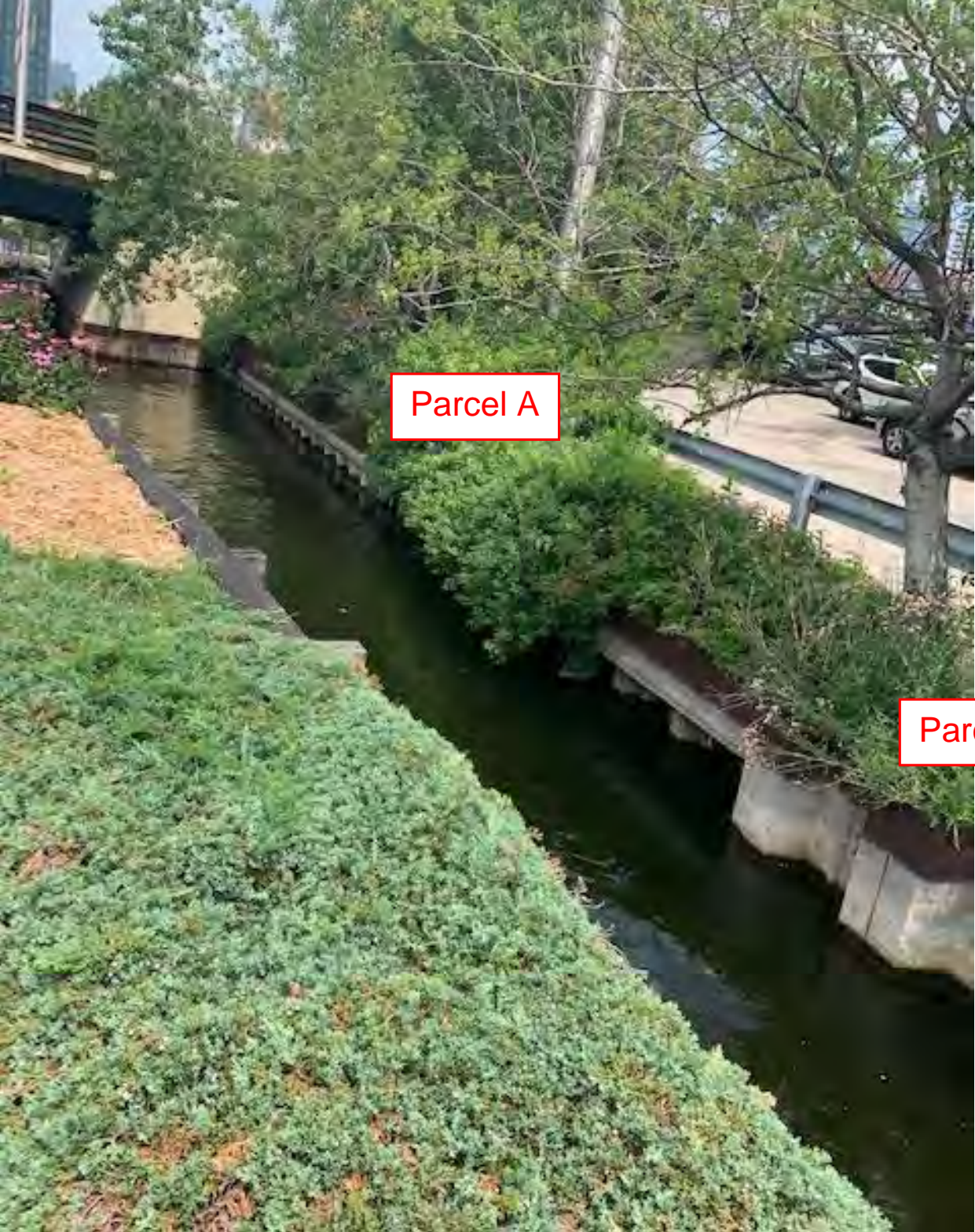
View from riverwalk of sheet pile dockwall transition of Parcel A and Parcel B.
