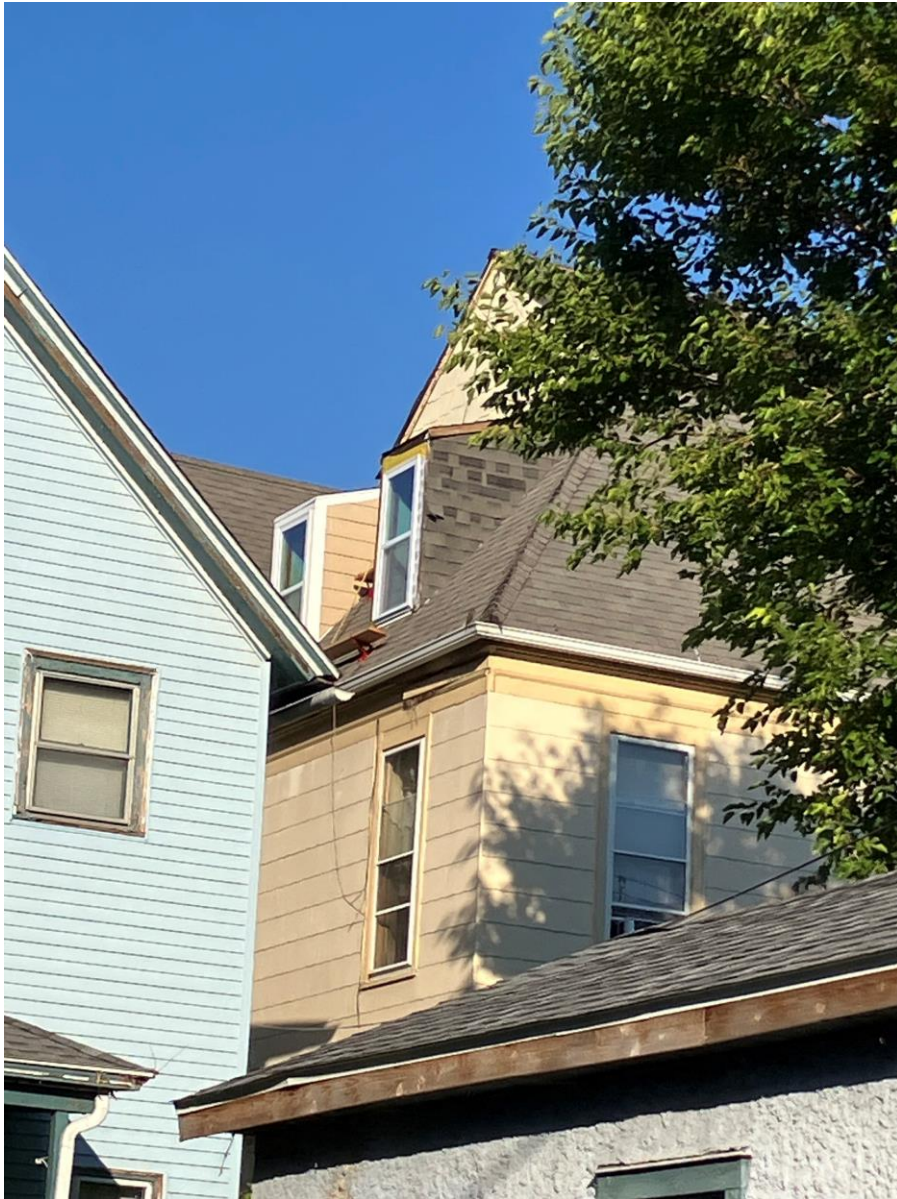
Replace asphalt siding on rear dormer to match the other dormer
