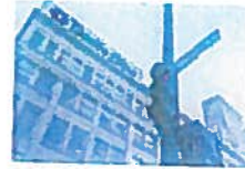
SCOTT FALCUS The Bon-Ton Stores offices are above the Boston Store at West Wisconsin Avenue and North Fourth Street.
