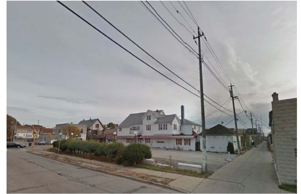
View Northeast from N. 37th Street
