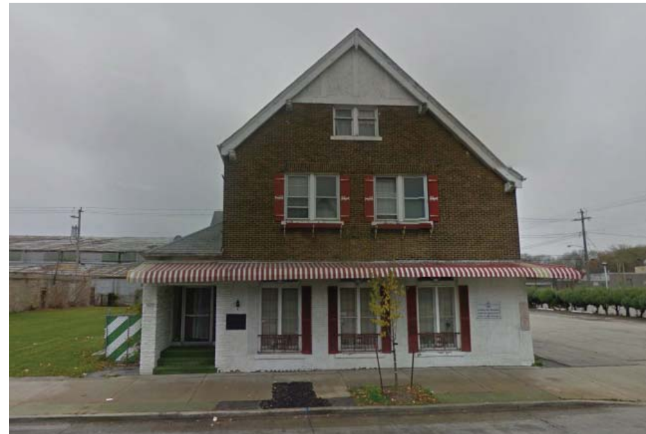
View of 3621 W. Villard Avenue
