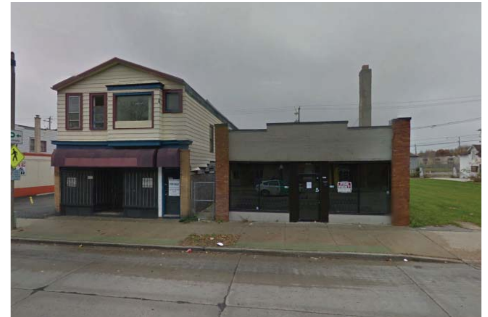
View of 3605-3611 W. Villard Avenue
