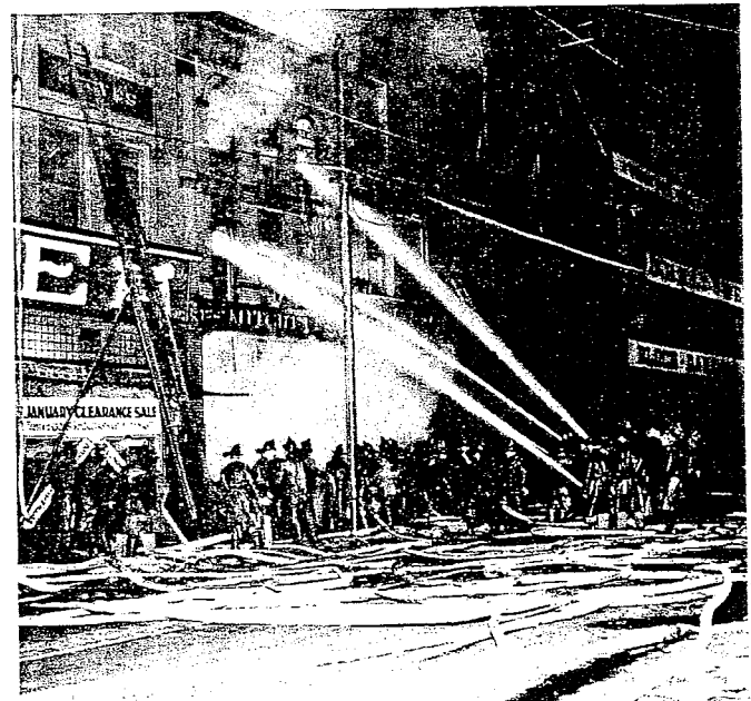
Fire on Milwaukee's south side, 1927.
