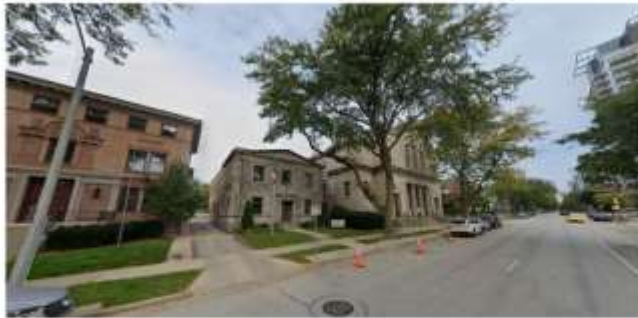
Existing Mexican Consulate Building - N Prospect Avenue
