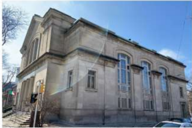
Existing 1451 N Prospect (Renaissance Place) - North Facade
