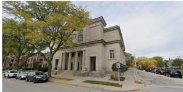
Existing Renaissance Place Building - N Prospect Avenue
