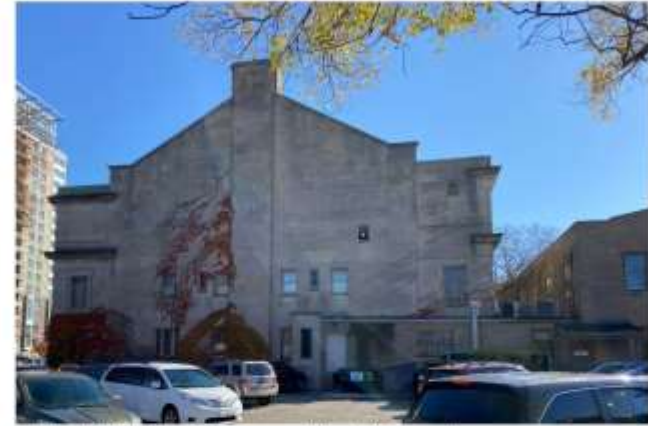
Existing 1451 N Prospect (Renaissance Place) - West Facade
