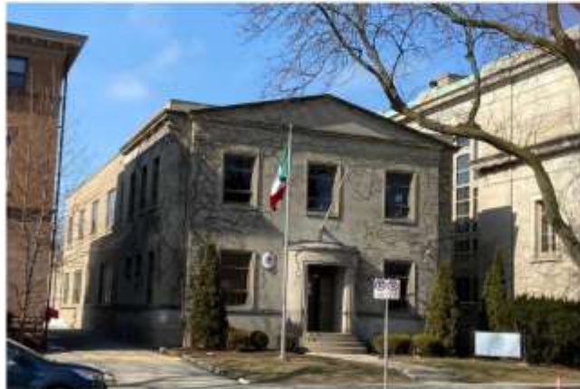
Existing 1443 N Prospect (Mexican Consulate) - East Facade & Landscape
