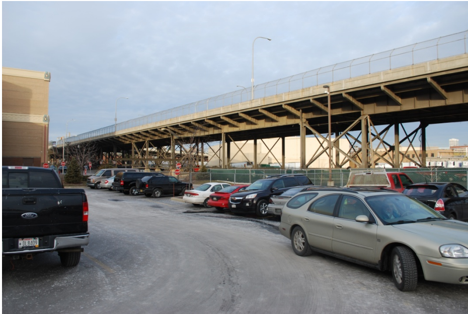
North East View from Parking Structure Site
