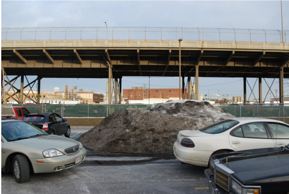
East View from Parking Structure Site
