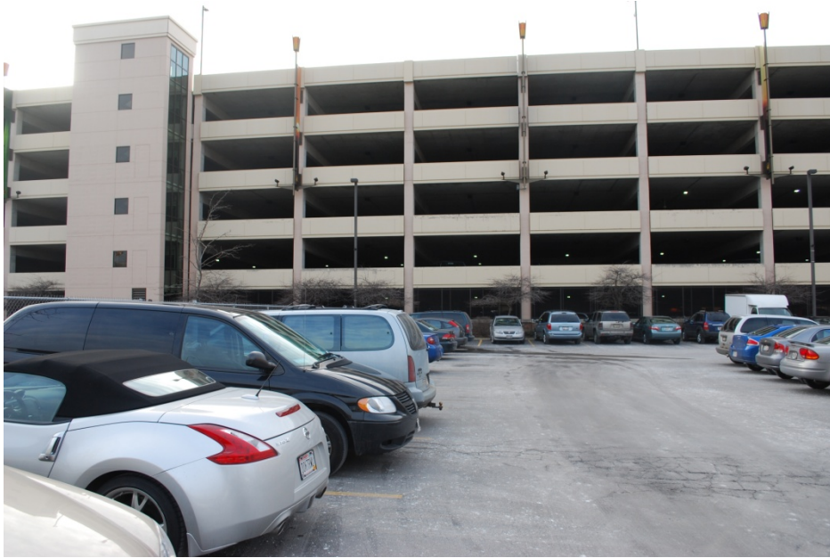
West View from Parking Structure Site
