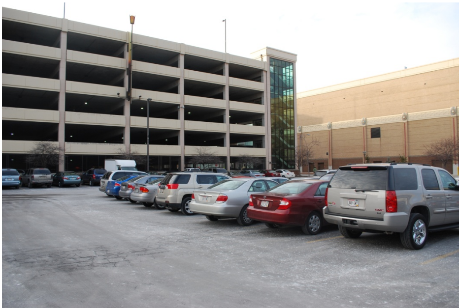
North West View from Parking Structure Site
