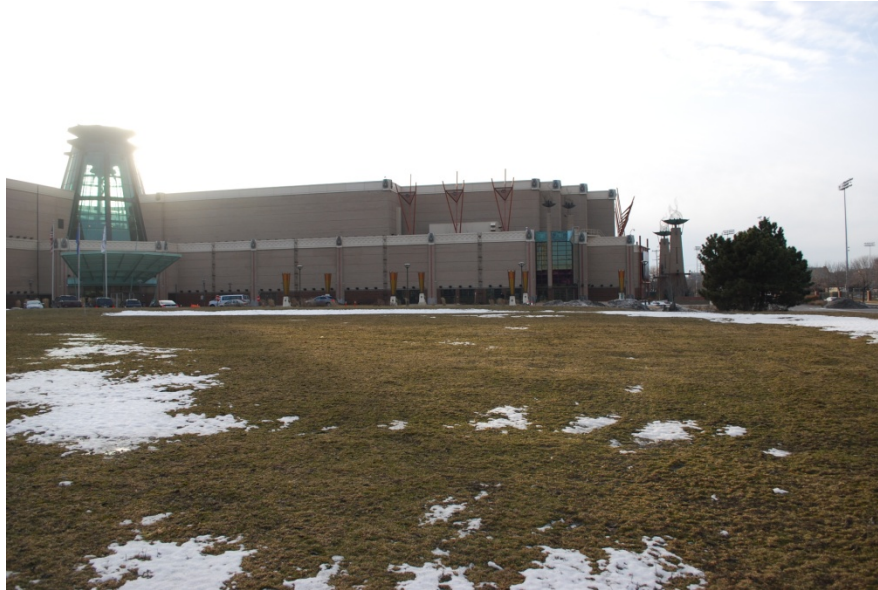
West View from Hotel Site
