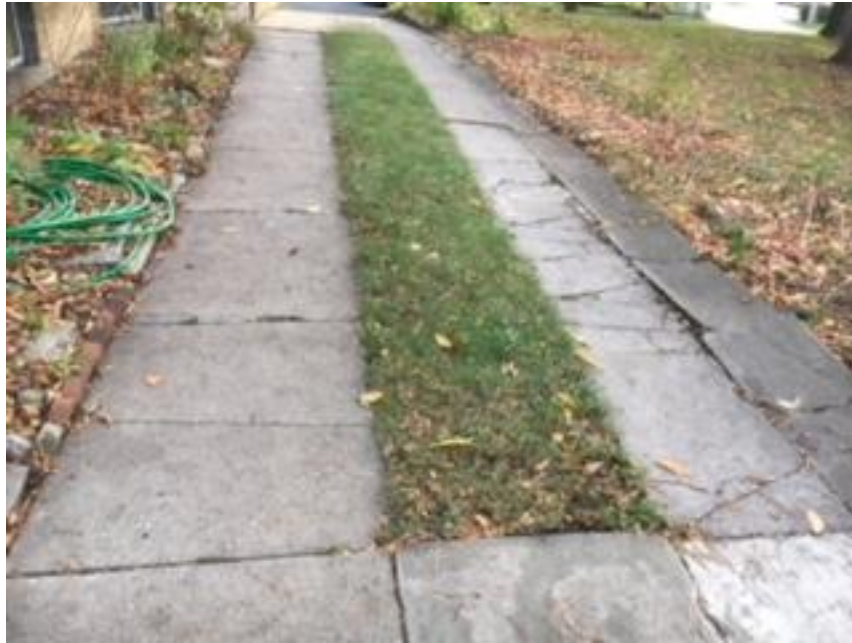
Photo above shows center section of driveway that will be replaced with concrete.
