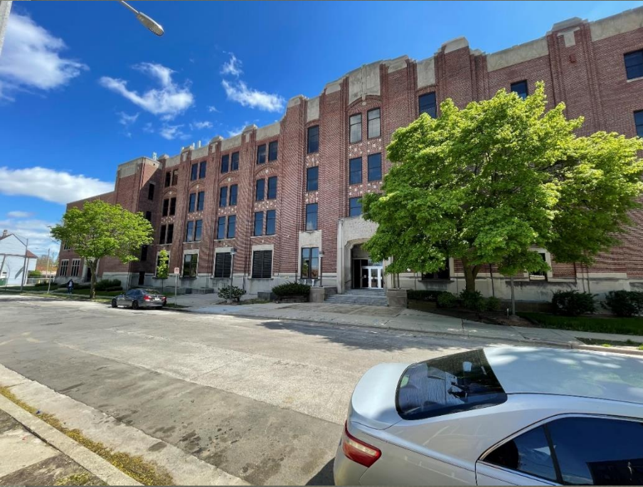
Wisconsin Telephone Toll Office 918 N. 26 th St 1929, Eschweiler & Eschweiler, architects
